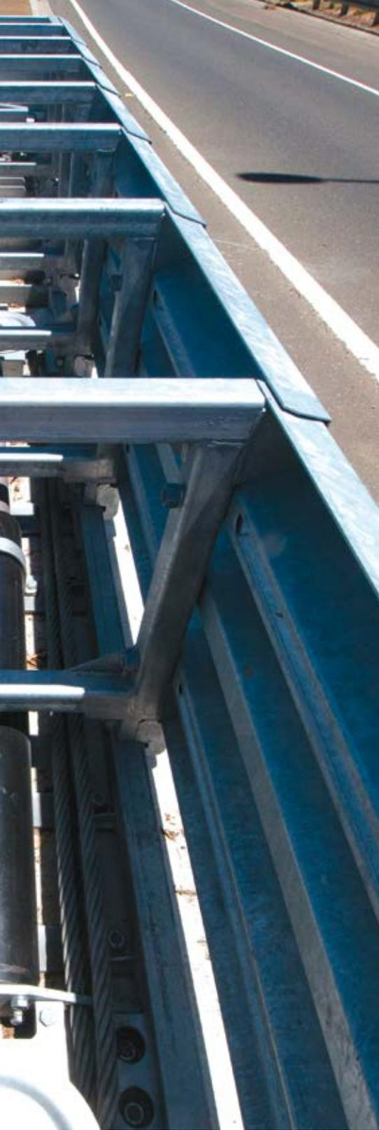
***“Unlike the old style attenuators, the SMART CUSHION attenuator rarely reaches maximum stopping resistance due to the interactive feedback nature of the system.”***
